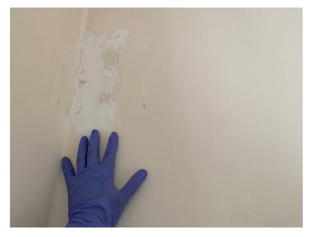
The rear chimney breast in the kitchen has been removed and it appears to be supported by a gallows bracket which is likely plaster boarded and skimmed over, I would advise making enquiries as to whether the necessary Building Regulations consents were in place in this regard and also the necessary Party Wall permissions and consents in regard to the property that this chimney breast adjoins.
