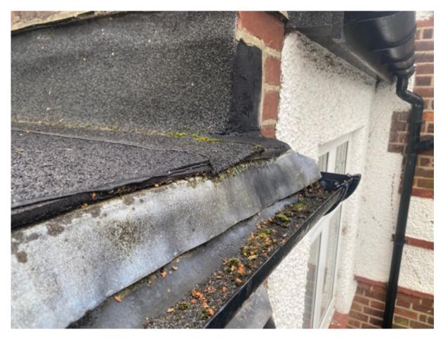
The gutters towards the rear of the ground floor extension are showing signs of moss growth and are unlevel throughout and I suspect in periods of heavy rain this could likely be spilling onto the fascia and rear extension itself.
