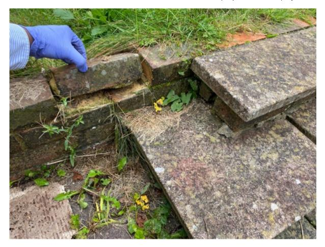
Towards the front of the property the boundaries to the left and right are set out by a single skin brick construction wall.
