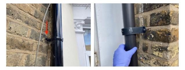
To the rear of the property the gutters are uPVC half-moon type. The downpipe towards the rear flank is detached from the wall. The clip itself has completely fallen away and this will need to be re-secured.
