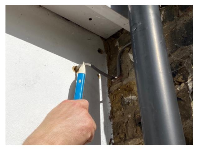
As previously advised, I would suggest that these are correctly installed and trunked in or alternatively, run internally to avoid a health and safety issue. It is worth noting that within the property there are a number of electrical sockets which are installed in unconventional places and at unconventional heights such as the flank of the chimney breasts.
