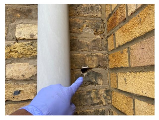
It is also worth noting that on the rear wall of the rear addition there is a drilled pole through the lower right corner whereby a wire is protruding and then running back into the flank wall of the kitchen itself.
