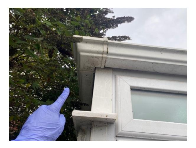
Towards the front of the property the gutters are uPVC half moon type. These appear to have been recently installed. All gutter clips were intact and neatly spaced.
