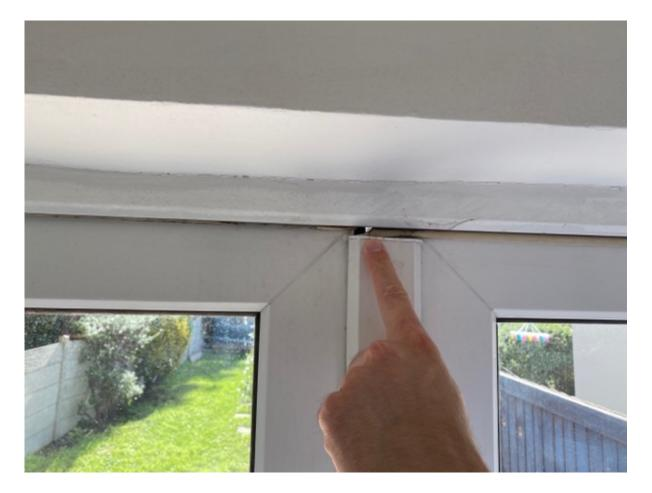
The doors will need to be adjusted to ensure that there is a weatherproof seal to their perimeter thereby stopping pests and weather from penetrating the internal parts of the property.
