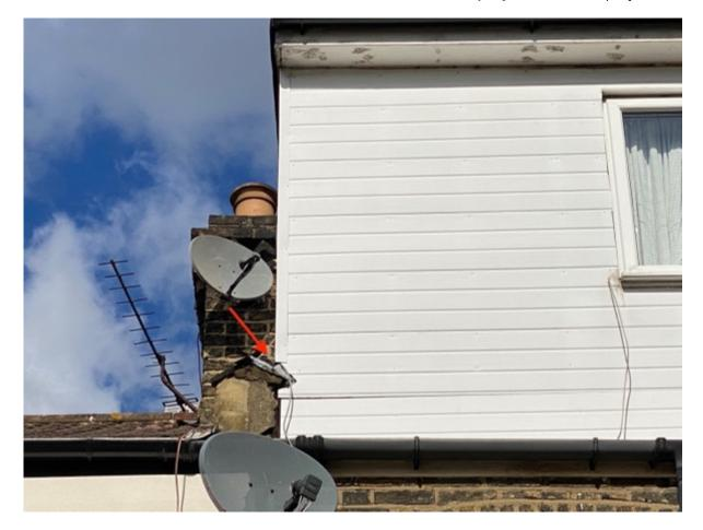
Generally speaking, this is a poor installation, and the conventional way would have been to remove the ridge tile and have a lead flashing dressed onto the party parapet wall itself with some form of considered final finish.
