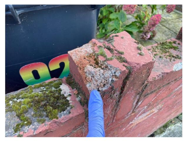
The boundary wall towards the front of the property adjoining the street is of the same single skin brickwork construction with bricks suffering from spalling and weather ingress intermittently throughout.
