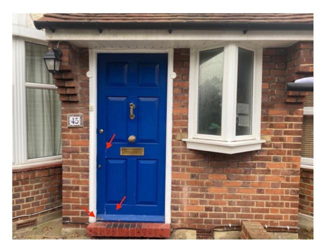
The front door is a uPVC double-glazed type, when the door opens and closes, the latch does not catch which means that the door needs to be manually locked internally via lifting the handle and turning the deadbolt.
