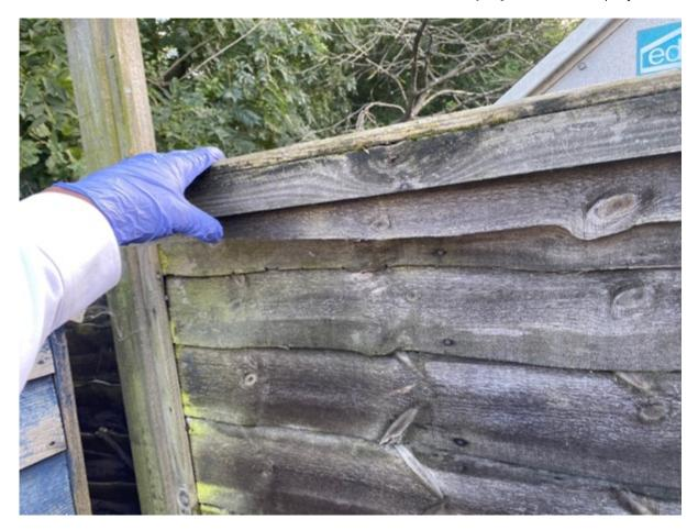
The fence panels themselves have completely failed and are significantly suffering from weather ingress, these will need to be replaced in the immediate future.
