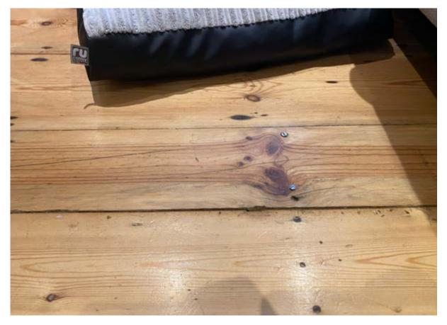
To the ground floor, the central wooden board, approximately 2.5m from the junction of the entrance, has been screwed down, and the screws themselves were sitting proud from the ground.
