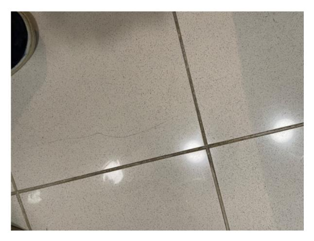
The ceramic tiles within the bathroom have cracked. Furthermore, the grouting has popped away intermittently.
