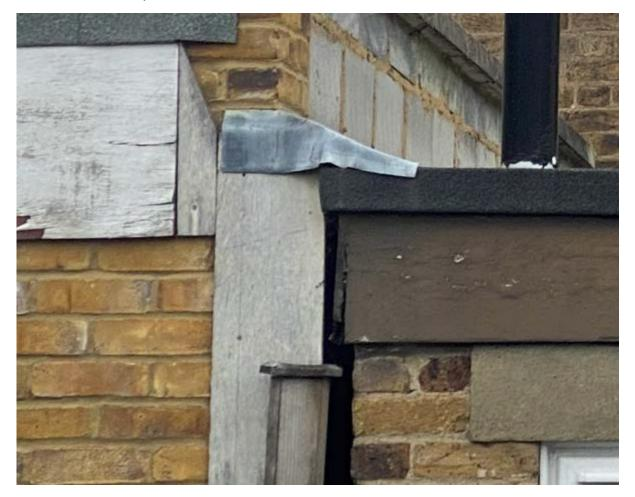
The roof to the rear extension, the fascia board towards the flank of the property itself, where it adjoins the semi-detached property, is showing signs of weather ingress and the fascia boards themselves are also showing signs of blistering and peeling paint throughout.
