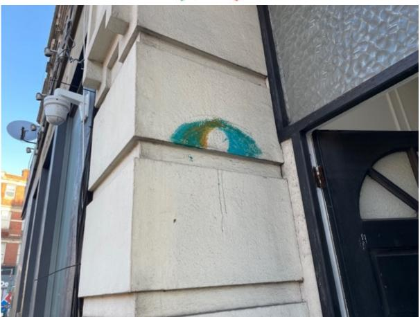
The front porch area has been maintained to a fair standard. However, there is an area of colouring noted to the left side of the opening. This should be cleaned away and repainted.
