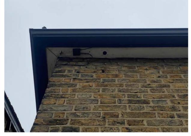
The rear rainwater gutter has been installed whereby it rests under the gutter to the other semi-detached property.
