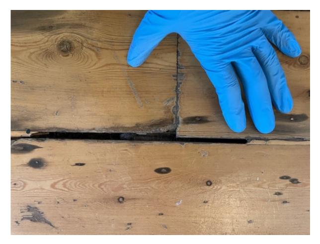
There are various gaps in between the floorboards, which will need to be sealed to avoid heat loss, dust build-up and pest infestation.
