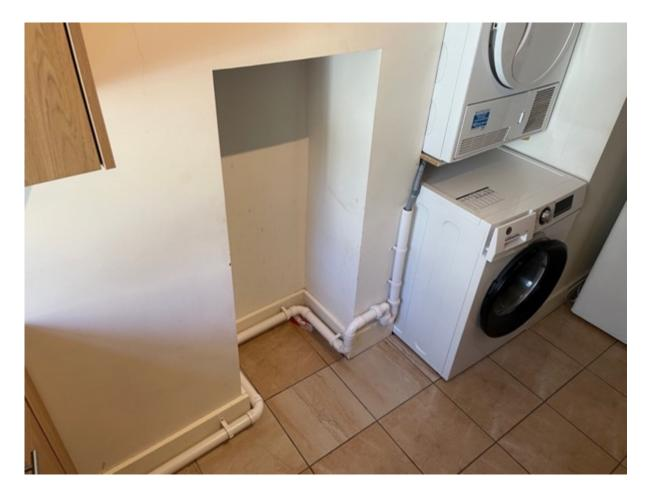
The washing machine waste feed pipework has been mounted to the wall. This is unconventional. You may want to consider having this reconfigured.
