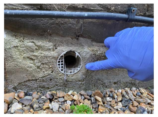
There appears to be a number of retro-fit circular core drilled air vents that have been inserted into the front and flank walls of the property.
