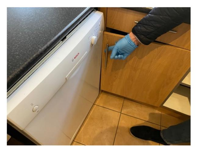
The cabinet door to the underside of the sink binds against the dishwasher. To address this, you can either install a smaller door and larger plinth or relocate the dishwasher.
