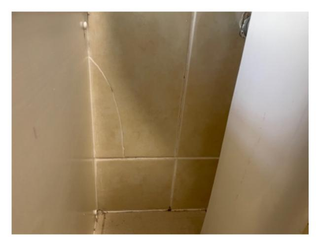
Some tiles to the perimeter of the bathroom have cracked. Unfortunately, there is no easy way to address this, and the tiles will need to be replaced.
