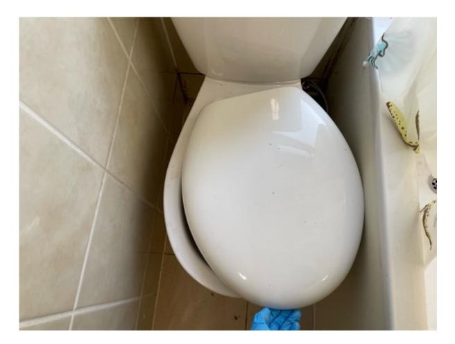
The toilet seat has come loose from its fixture and will need to be firmly fixed back in place.
