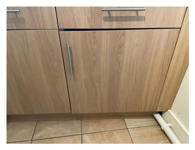
A number of the fitted cabinet doors had dropped from their fixings. To address this, the hinges would need to be adjusted.
