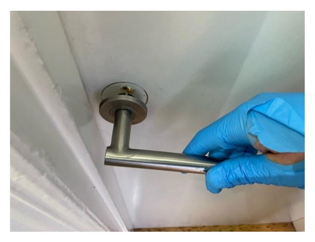
All internal doors are of timber type. The majority of the door handles are defective, with the bathroom door being made good to a DIY standard.
