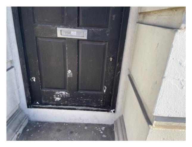
The main entrance door is of a timber type, and could benefit from repainting. However, the door was operational.
