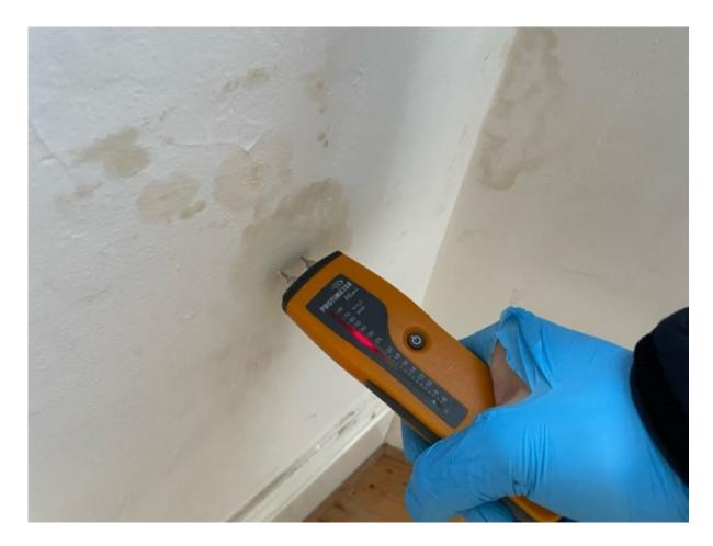
A further area of staining was noted within the left front room to the bay area. When probed with the Protimeter, I also obtained a red reading which confirms the presence of moisture.
