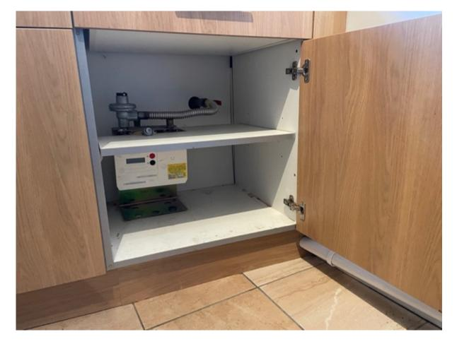
I was able to locate a gas meter to the underside of the sink. This is an unconventional location for a gas meter.
