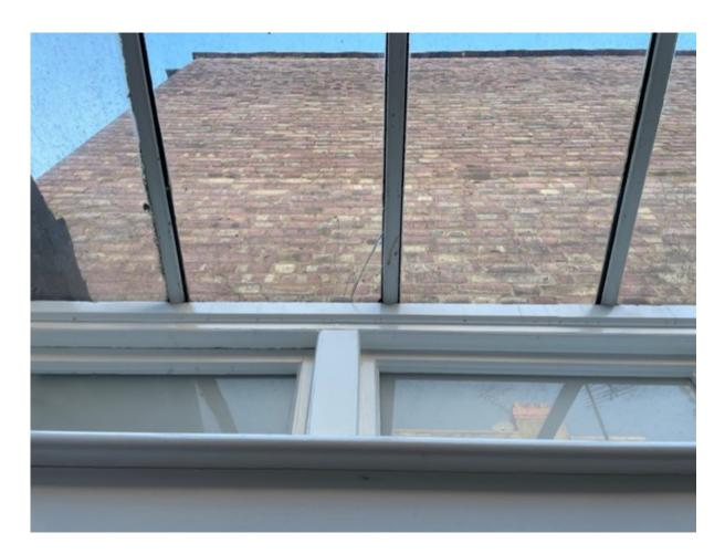
The glazed roof of the reception area has cracked. Unfortunately, there is no easy way to address this, and the defective glazing will need to be replaced.
