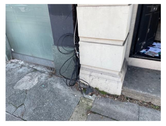
To the flank of the property, there are loose wires from the neighbouring property, which are protruding onto the demised area of the subject property. These should be clipped away neatly.
