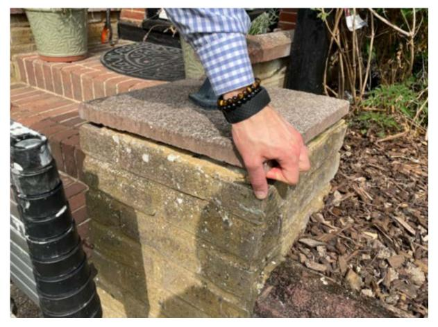
There is a brickwork London stock single skin construction wall, this is significantly weathered. While the wall does have four respective buttresses, which given its length will provide sufficient support. It is showing signs of significant weather ingress throughout, lichen and moss growth throughout, and will likely require some maintenance and repair immediately.
