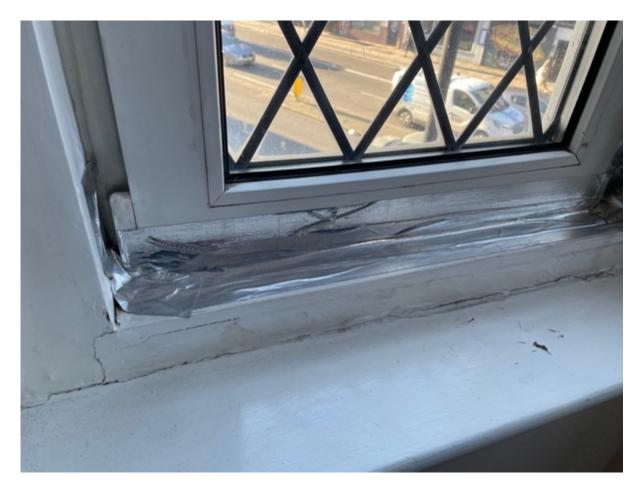
Intermittently, glazing has blown. Handles are defective and non-operational. Duct tape has been utilised to seal junctions, which is unconventional.
