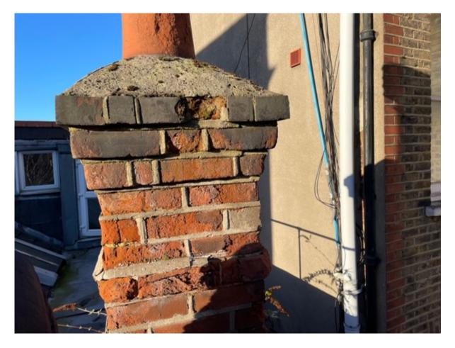
There are three more stacks visible from the roof terrace at the rear of the property. All stacks are displaying spalling, missing areas of pointing, defective flaunching, cracked and spalling pots, and have reached the end of their useful life.
