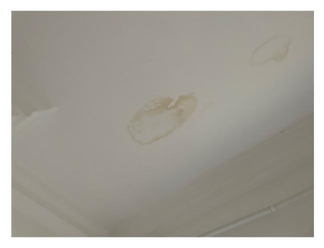
There are also general areas of staining, flaking and blistering on the ceiling surfaces. This is to be expected, given the current condition of the external roof coverings, causing saturation to the plaster, through moisture and water ingress.
