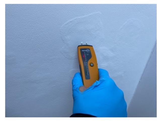
In various areas within the property, there was various blistering and flaking to the plaster finish, predominantly due to the aforementioned failed roof coverings.
