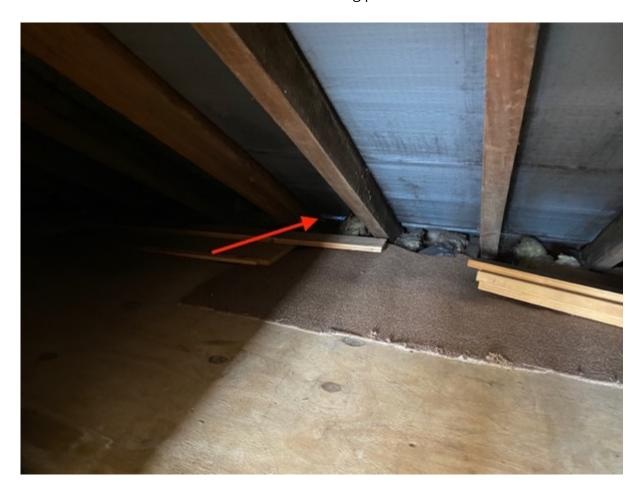
This could result in pest ingress and weather ingress and therefore I would advise that a competent roofer inspect this area to ensure that the tiles are properly laid and level throughout.
