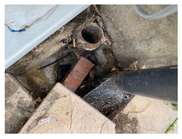
This is a slightly unconventional finish and generally speaking, they should be covered with a grate or drain cover.
