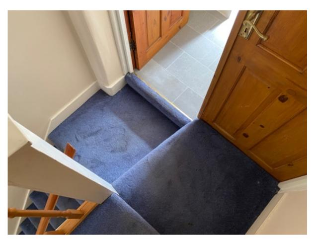
This is relatively unconventional and generally speaking, when development works do take place to a property, Architects tend to design around and avoid this type of issue as they can be tripping hazards and generally are quite awkward to work around and I would therefore suspect that the works that have taken place were poorly considered at the time of their conception and that could be an indication that the necessary statutory consents could not be in place.
