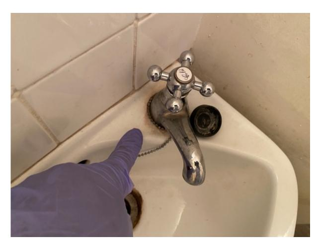
The property benefits from mains fitted water in both the kitchen and bathroom areas. At the time of the inspection the shower was tested and there was no water running as were the taps which likewise had no water running through them.
