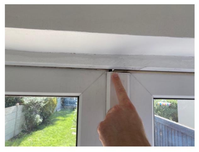
The doors will need to be adjusted to ensure that there is a weatherproof seal to their perimeter thereby stopping pests and weather from penetrating the internal parts of the property.
