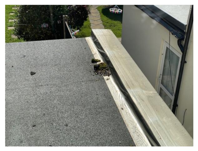
Flashband, generally speaking, has a very short lifespan and ideally this would have been done with a lead flashing which increases the longevity of the abutment itself.
