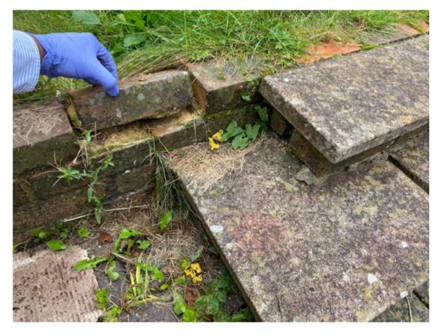
Towards the front of the property the boundaries to the left and right are set out by a single skin brick construction wall.
