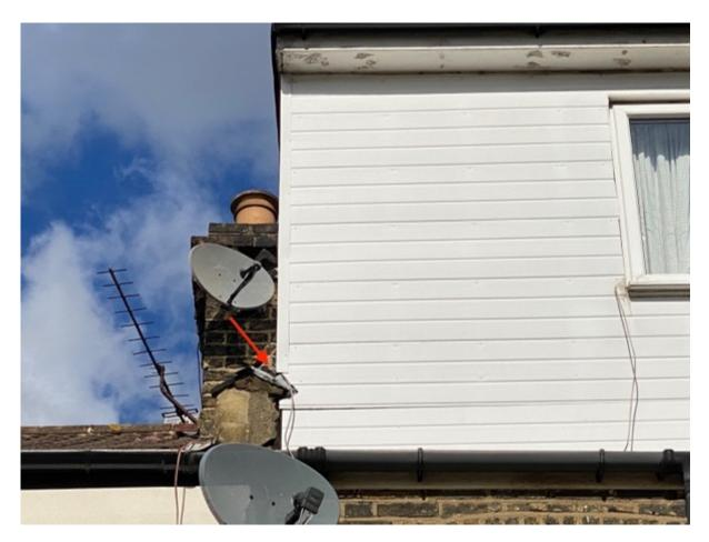
Generally speaking, this is a poor installation, and the conventional way would have been to remove the ridge tile and have a lead flashing dressed onto the party parapet wall itself with some form of considered final finish.
