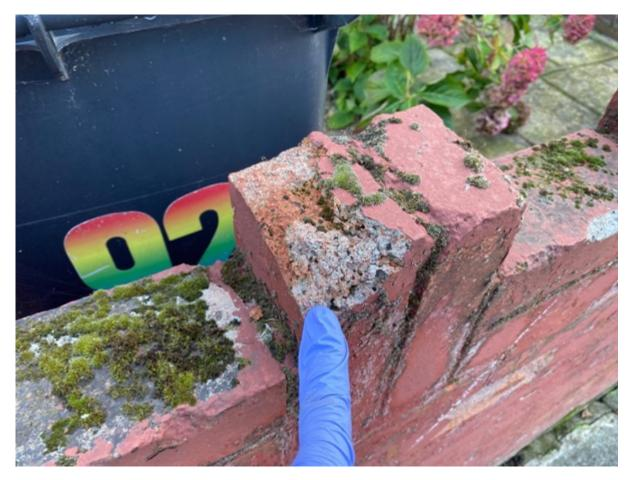
The boundary wall towards the front of the property adjoining the street is of the same single skin brickwork construction with bricks suffering from spalling and weather ingress intermittently throughout.
