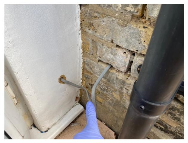
This would not be Health and Safety or Building Regulations compliant as the wire can be pulled and moved, and I would advise that this is either boxed in, trunked in or the conventional wires are run through the internal voids of the property.
