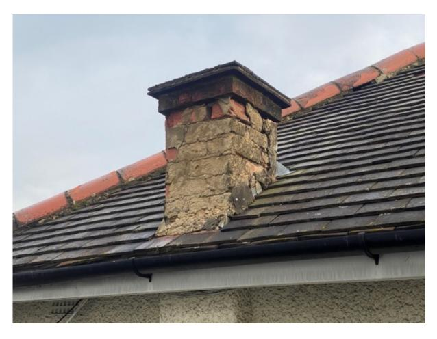
The chimney stack is of brickwork London stock solid construction. There are a total of eight pots on the stack shared with the adjoining property.
