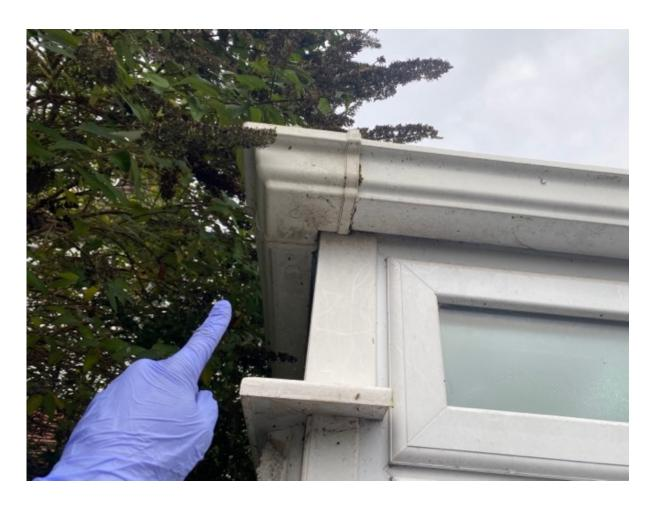
Towards the front of the property the gutters are uPVC half moon type. These appear to have been recently installed. All gutter clips were intact and neatly spaced.
