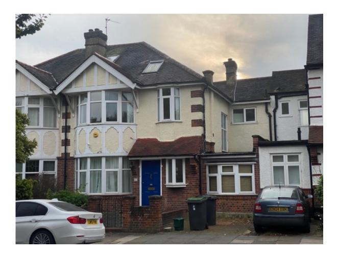
The property is a solid brick London stock construction beneath a pitched roof. The roof is covered with concrete interlocking tiles.
