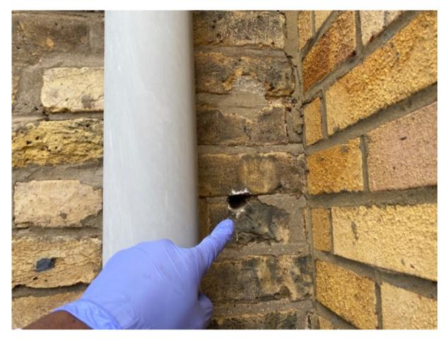
It is also worth noting that on the rear wall of the rear addition there is a drilled pole through the lower right corner whereby a wire is protruding and then running back into the flank wall of the kitchen itself.
