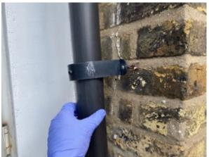
To the rear of the property the gutters are uPVC half-moon type. The downpipe towards the rear flank is detached from the wall. The clip itself has completely fallen away and this will need to be re-secured.
