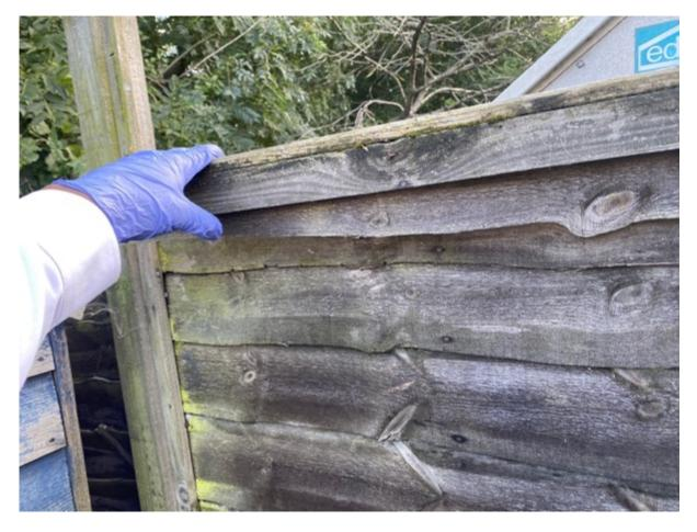
The fence panels themselves have completely failed and are significantly suffering from weather ingress, these will need to be replaced in the immediate future.
