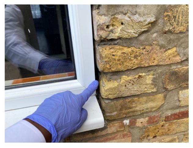
These should be filled with a neat bead of cement or neat bead of mastic to ensure weather and pest ingress is not able to penetrate the internal parts of the property.
