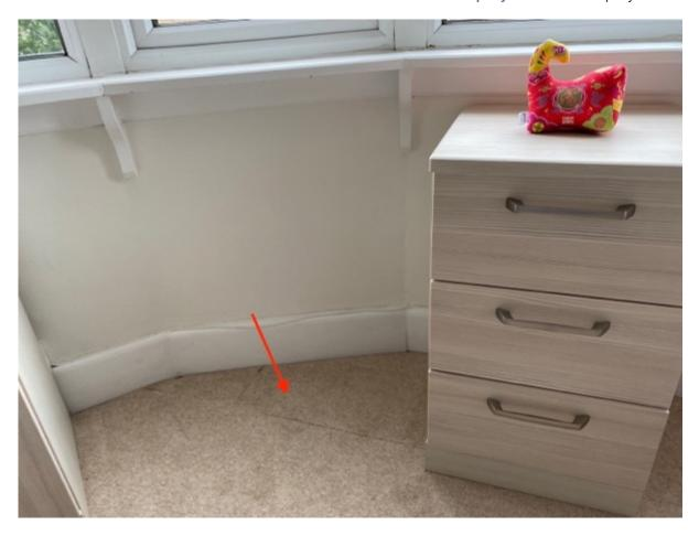
Within the first-floor front bedroom the front of the bay there are a number of different carpet joins noted and generally speaking, for a room of this size there should have been one continual sheet of carpet which would have then been cut to size.
