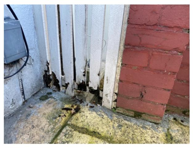
The boundary walls themselves, when tested with a firm lean, do move and therefore you may want to budget into the maintenance costs in the near future to replacement and upgrade of these respective walls.
