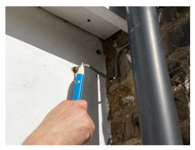
As previously advised, I would suggest that these are correctly installed and trunked in or alternatively, run internally to avoid a health and safety issue. It is worth noting that within the property there are a number of electrical sockets which are installed in unconventional places and at unconventional heights such as the flank of the chimney breasts.
