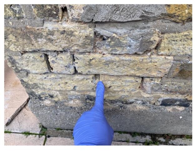
Generally speaking, this is usually a sign that the pointing that has been done is insufficient and I suspect in due course defective pointing will need to be raked out and filled to ensure that there is a sound weather break between the external areas of the property and the internal walls themselves.
