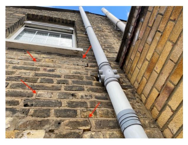
These types of cracks are relatively normal and generally speaking the gap between windows at ground and first is a soft spot and is susceptible to movement.
