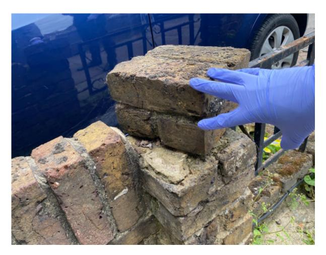
The central pier/buttress, the upper section of the brickwork is loose when tested and is not held in place firmly. This is a danger and will need to be bedded in with suitable cement.
