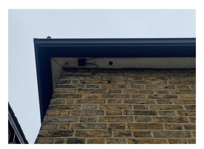
The rear rainwater gutter has been installed whereby it rests under the gutter to the other semi-detached property.
