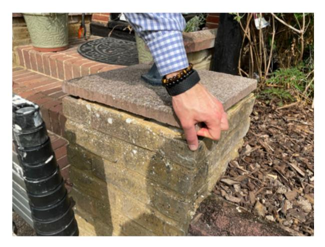
There is a brickwork London stock single skin construction wall, this is significantly weathered. While the wall does have four respective buttresses, which given its length will provide sufficient support. It is showing signs of significant weather ingress throughout, lichen and moss growth throughout, and will likely require some maintenance and repair immediately.
