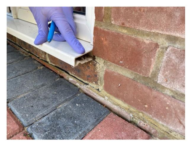
Some of the windows have trickle vents which is favourable as it ensures that airflow can naturally move through the property without windows being open, reducing condensation build up within the demise itself.
